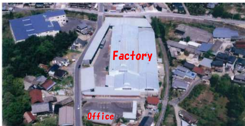
The aerial photo of Gifu Manufactory
